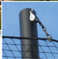
Coated galvanized steel cable across top minimizes "net sag".
